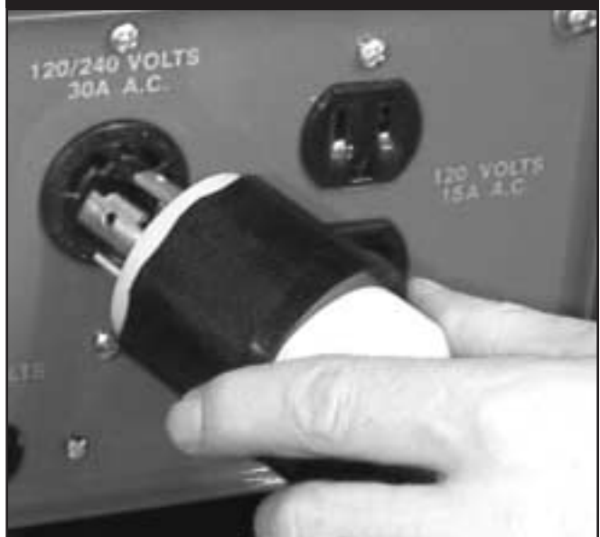
Figure 23 — Align Connectors at Generator
