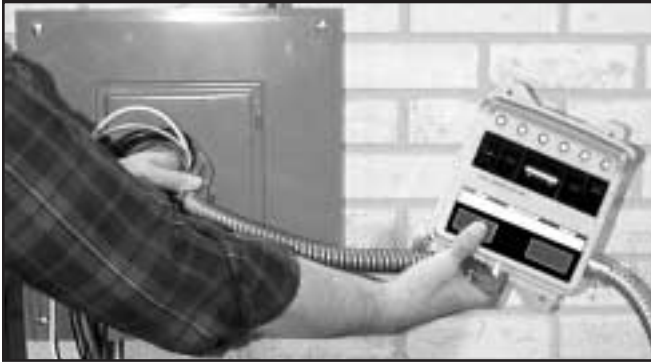
Figure 3 — Planning Switch Location
