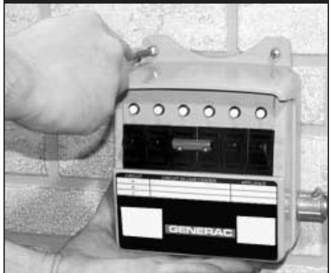
Figure 5 — Anchoring Load Manager™ Switch
